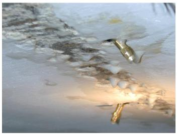
TamPur 150 MDI is a single component hydrophilic polyurethane in combination with polyether polyols. It only reacts when it comes in contact with water and forms a flexible polyurethane seal.
